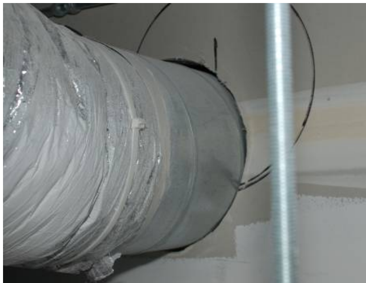
Figure 3-6 Sealing Penetrations
