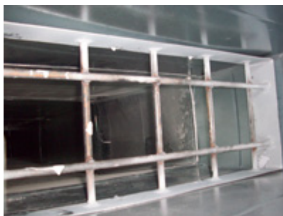
Figure 3-7 Bars on Penetration
